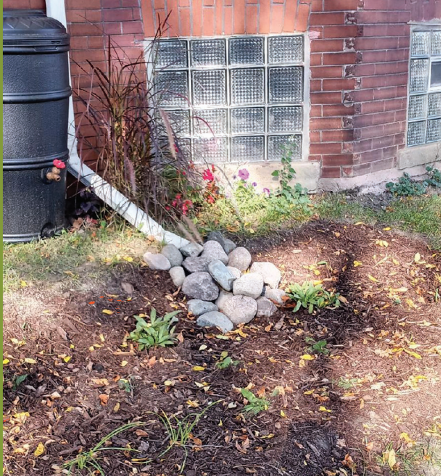
MILWAUKEE GREEN SUMMER PROJECT
